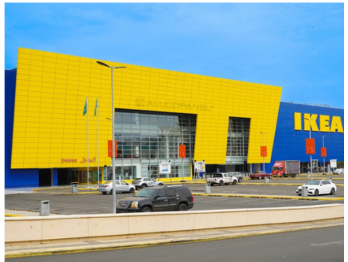
IKEA, Althalia Street, Jeddah, KSA Product used: Alucopanel® FR Volume: 12,500 SQM
