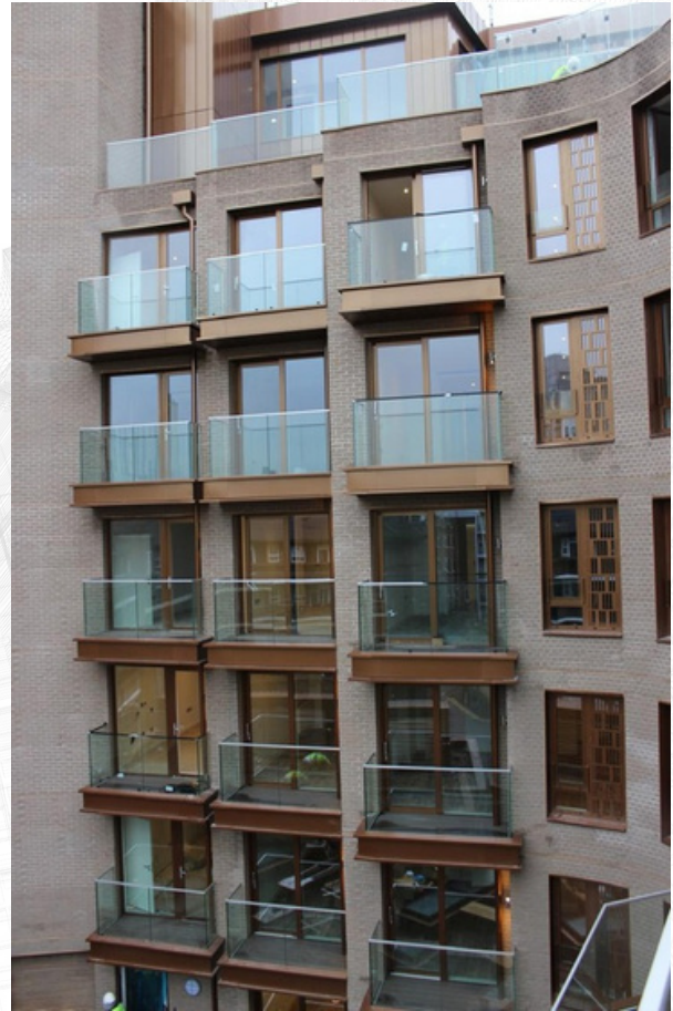
Lambeth High Street Apartment M-SPAN BetterFIX M12 profile used
