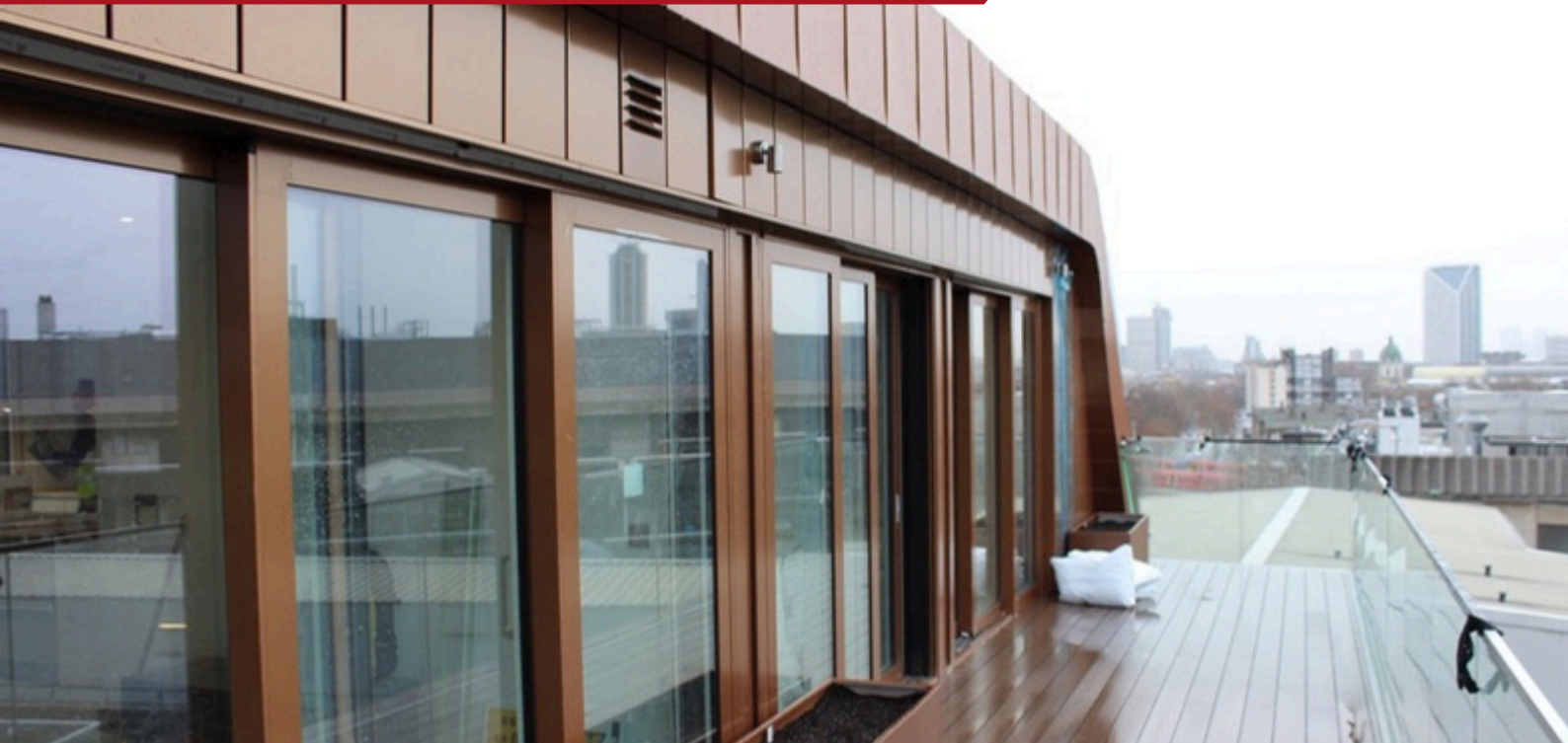
Lambeth High Street Apartment M-SPAN BetterFIX M12 profile used
