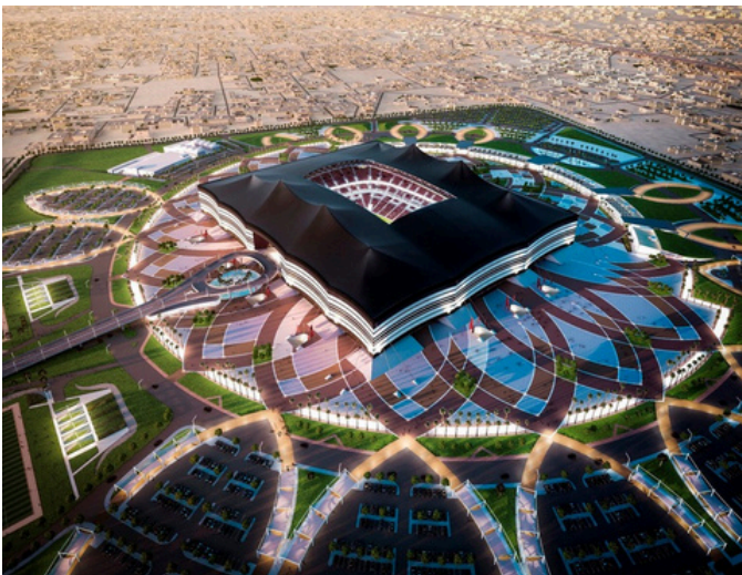
Al Bayt Stadium in Qatar Product used: Fire-safe Alucopanel® FR Volume: 15,000 SQM
